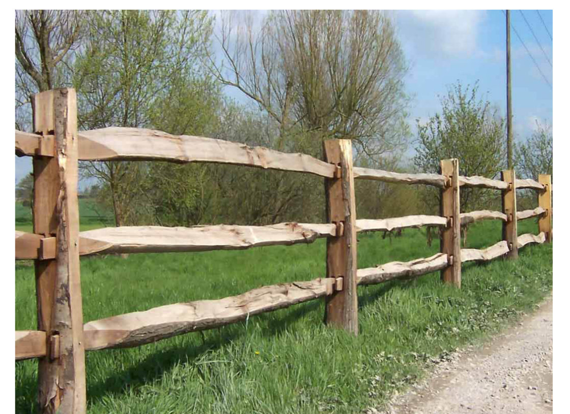
Image 1 - 1.2m Timber Cleft Rural Fencing
