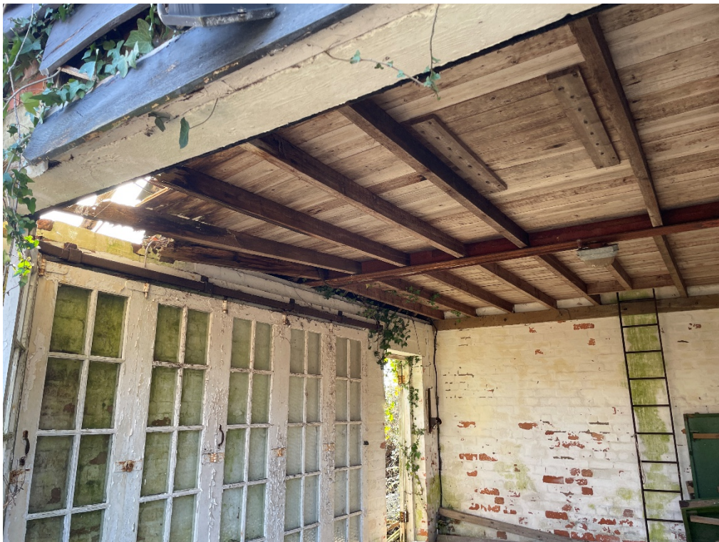
Photograph 4 – One of two outbuildings to front of property
