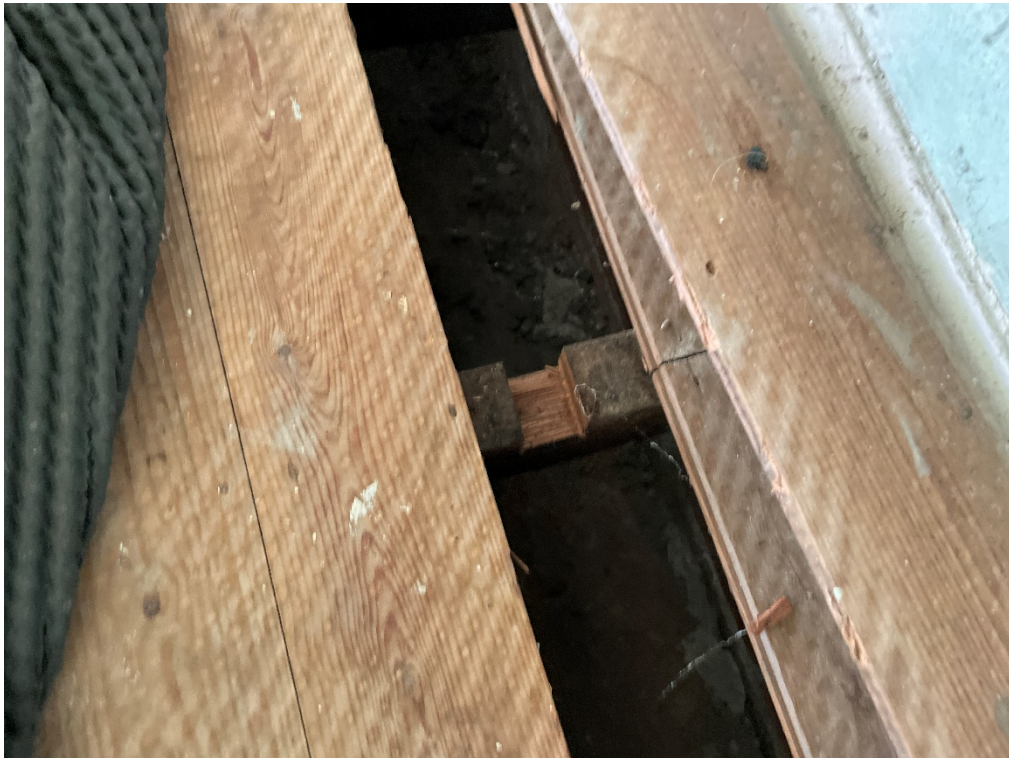
Photograph 9 – Suspended ground floor timber joists
