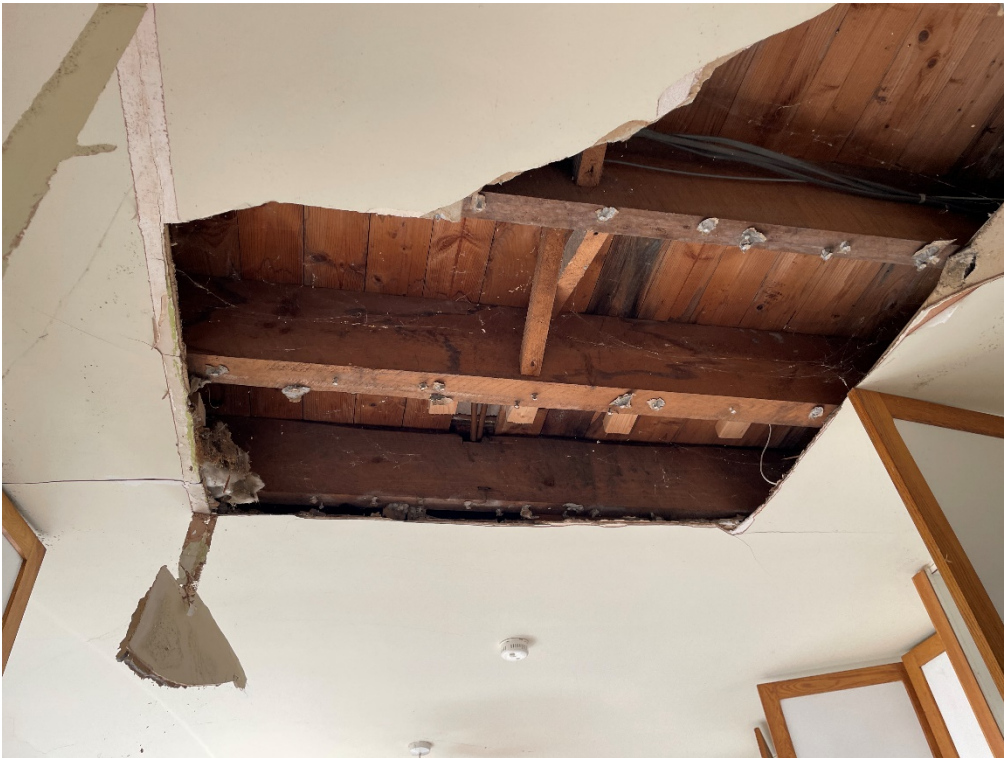
Photograph 8 – Exposed first floor timber joists
