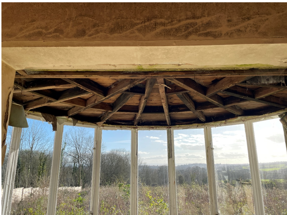
Photograph 6 – Rear sun room timbers
